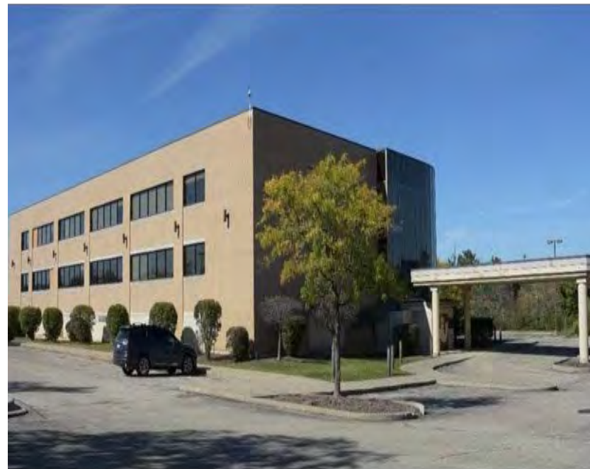
Future site of the VACWC; 1300 Copperfield Ave Joliet, Illinois
